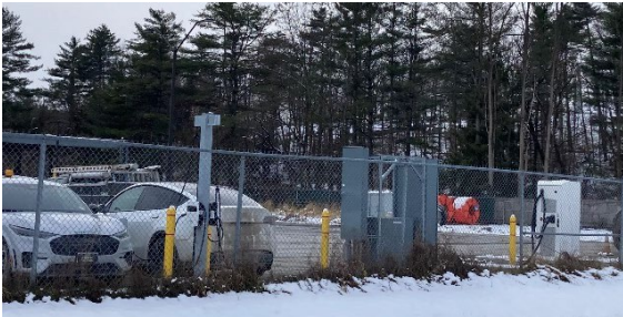
34 Example 1: EVSE behind a fence owned by a public utility for their exclusive use.
